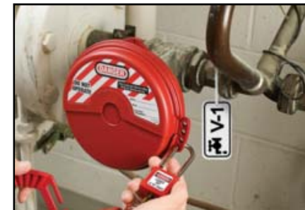
V-1 Tag Identifying Valve Lockout Point
