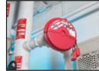
Gate Valve Lockout
