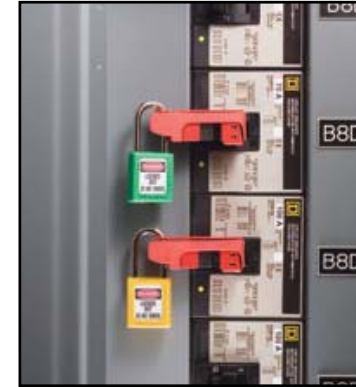
Circuit Breakers Locked Out to Prevent Accidental Energization
