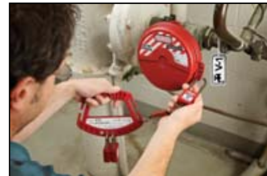
Worker Locking Out Gate Valve Using S125
