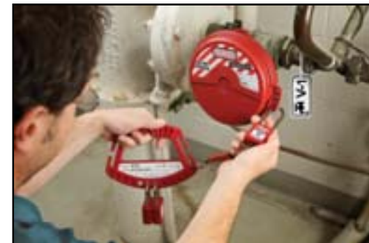
Worker Locking Out Gate Valve Using S125
