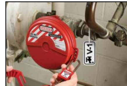
V-1 Tag Identifying Valve Lockout Point
